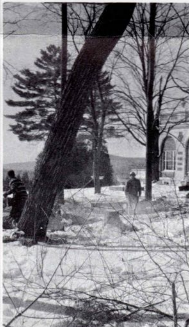
Tree clearing for the Seminary addition
