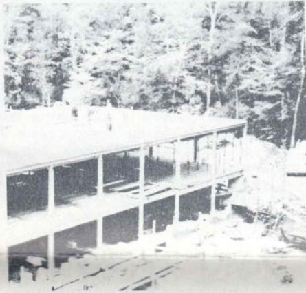
The workmen pouring the roof over dormitories of North-South Wing.
