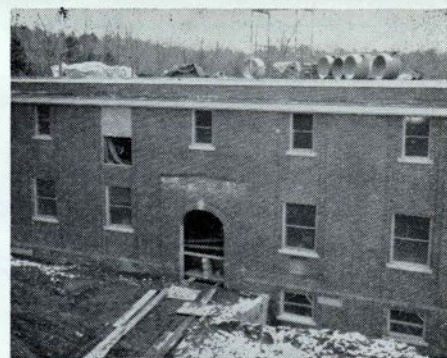
The front section is almost completed.
